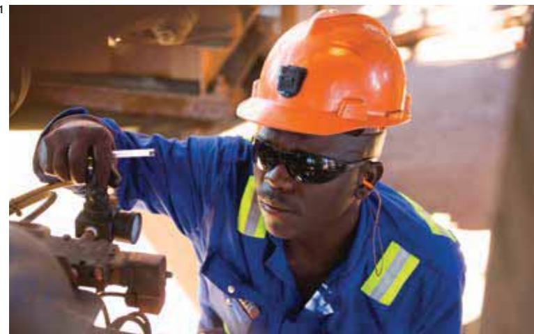
02 Fitters Laura Zuba and Bahny Motshabi work on a diesel engine in the newly completed vehicle workshop for mega class equipment at Sishen mine.
